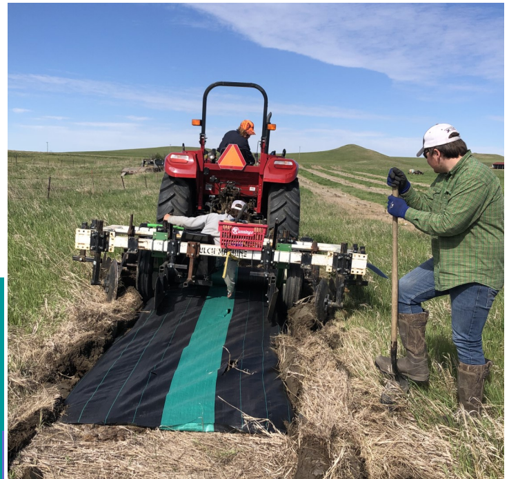
Tree Crew Laying Fabric
